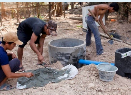
Workers installing the building blocks of a new latrine for a rural household. Photo: iDE
