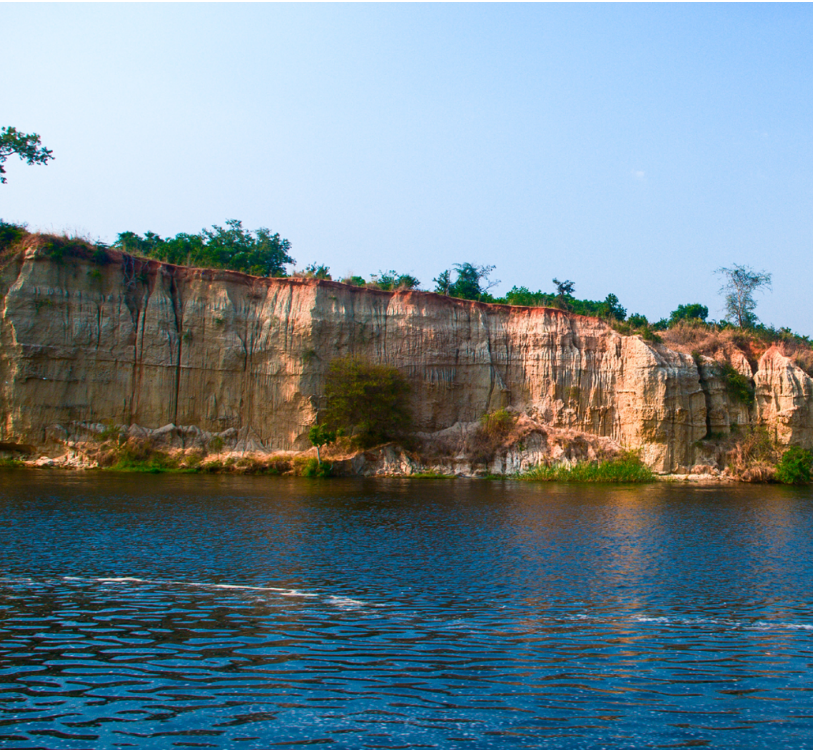
Nile bankment in Masindi, Uganda. Photo: Floschen/Creative Commons
